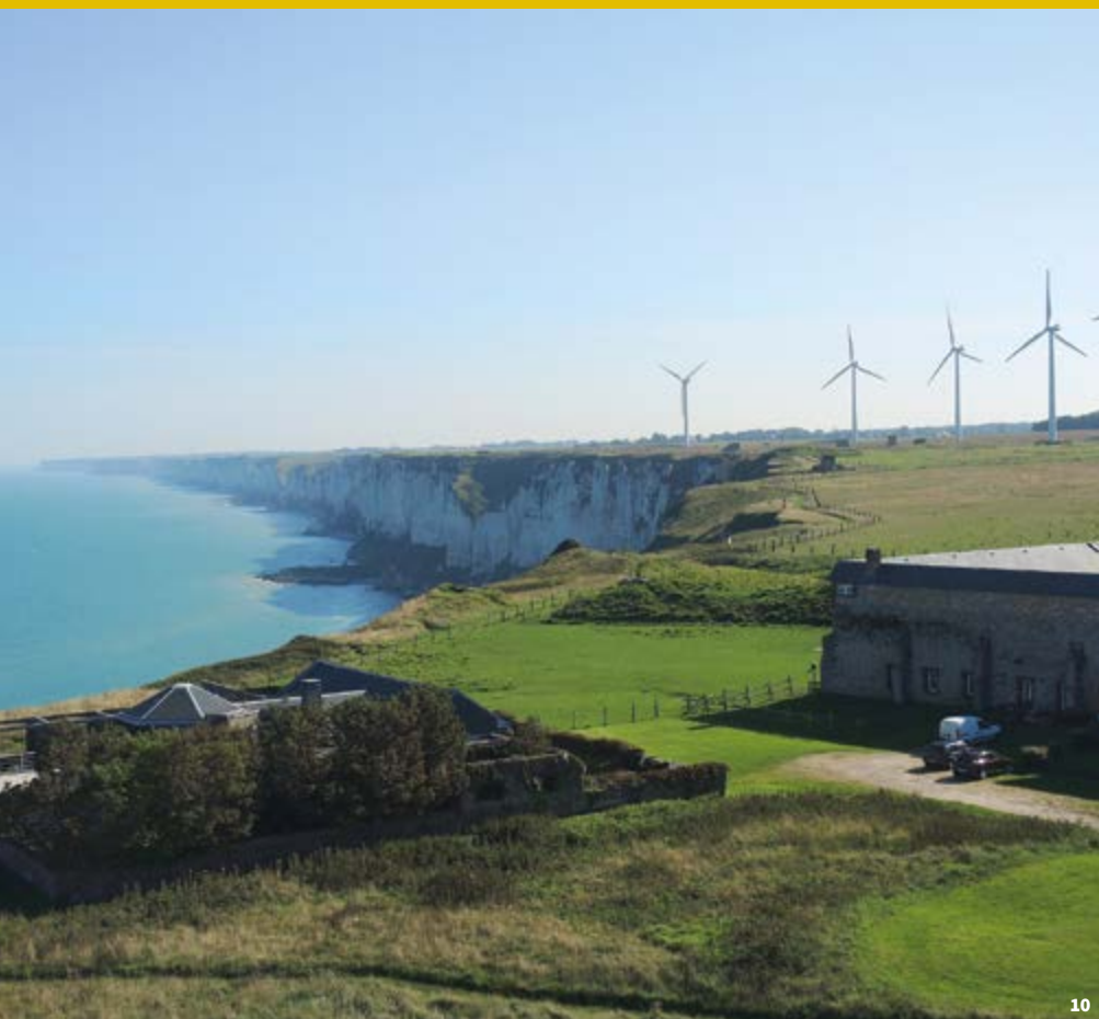
10. View of the windfarm from the cliff near Saint-Valéry-en-Caux
